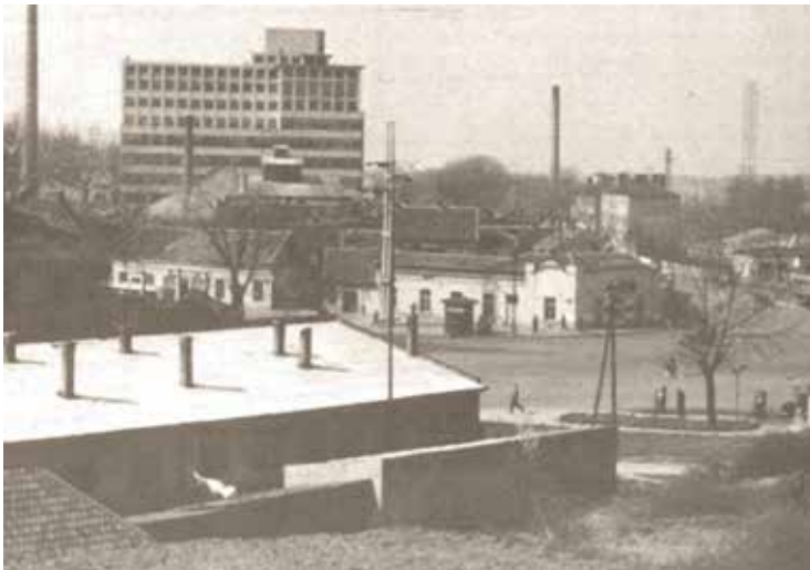
Fig. 5: The Mostar area with new industrial buildings in the beginning of 20th century (Source: https://www.google.rs/search?q=mostar,+beograd&rlz=1C1GGGE___RS544RS566&source=Inms&tbm=isch&sa=X&ved=0ahUKewjXq_-08q_NAhUBrRQKHe7kB7MQ_AUICcgB&biw=1366&bih=643#tbm=isch&q=Zbirka+kasine%2C+belgrad%2C+mostar%2C+razglednica&imgsrc=lxUEQZwqQYP7_M%3A ).
