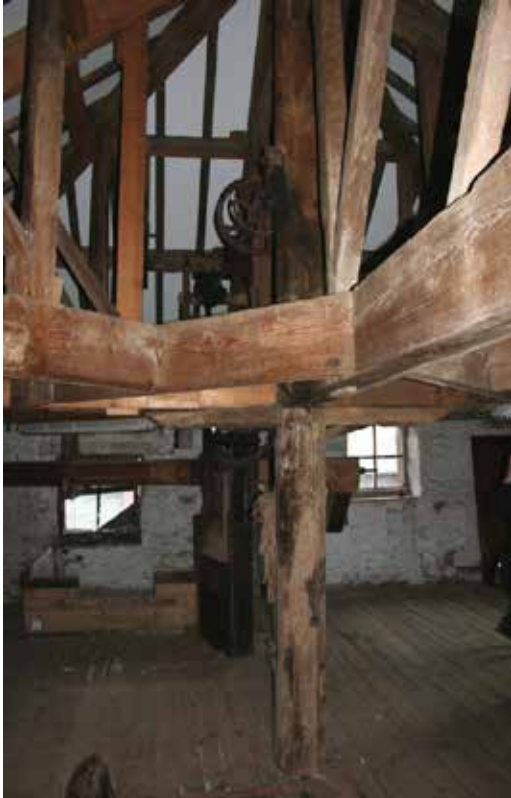
Fig. 13: Warwick Bridge Corn Mill (Cumbria) an early 19th C water powered corn mill, significant for its intact machinery and waterwheel (dated 1843) remained in operation until 1989, but has been on the Heritage at Risk Register since 1999 (15 years). The roof has been repaired by the owner but the overall condition is poor. Options for a more comprehensive restoration to secure a sustainable use by the North of England Civic Trust (NECT) are under discussion at the present time. NECT was awarded a grant of £1,379,300 (GBP) from the Heritage Lottery Fund (HLF) in June 2015 towards its ambitious £2 million (GBP) project to bring the building back into operation as a working mill and artisan bakery providing specialist courses in bread-making with associated crafts, and as a resource for learning in connection with the national school curriculum and accredited conservation courses. The building has been bought by NECT for this working project with the assistance of a low interest loan from the Architectural Heritage Fund (set up as part of the UK's contribution to the European Architectural Heritage Year campaign 1975 to assist such rescue projects). Work should commence in late 2015. Had this option not been realised the property has had the benefit of planning permission to convert the building to residential use, but this would have resulted in the loss of the machinery.
