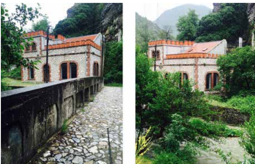
Fig. 2: Hydroelectric power plant "Prizrenasja", Prizren, photo Safete Veliu.
