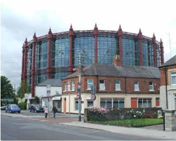
**Fig. 4:** Dublin Gasworks: Late nineteenth century gas holder was converted into a multi-storeyed apartment building in 2006.
