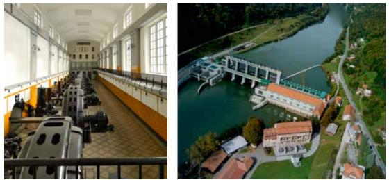
**Fig 3:** Heritage of industrial companies is an important part of their identity and a testimony to its tradition as the basis of their success. On the occasion of its 80th anniversary, the company Dravske elektrarne Maribor restored its former hydroelectric power plant Fala and converted it into the company's museum. Photo: Miran Kambič.
