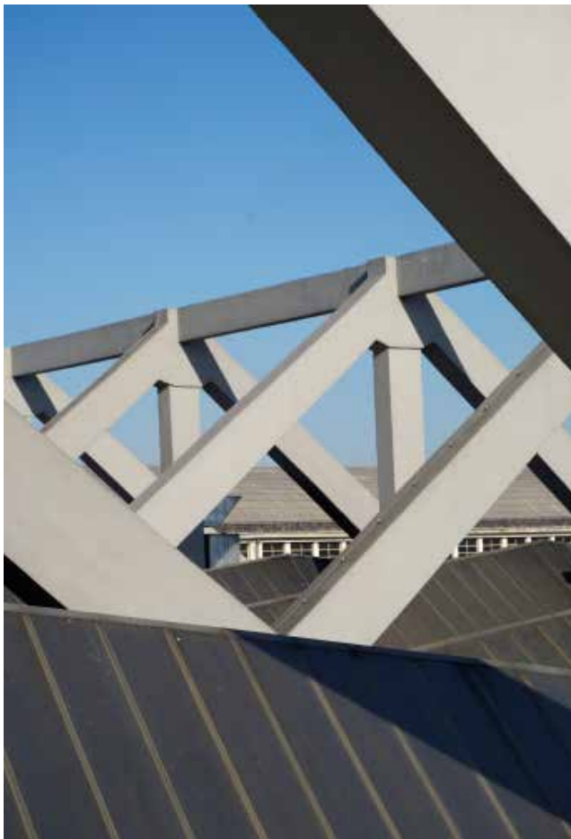
Fig 4: The suspended construction and roof structure of the metalworking plant. Photo: Miran Kambič.
